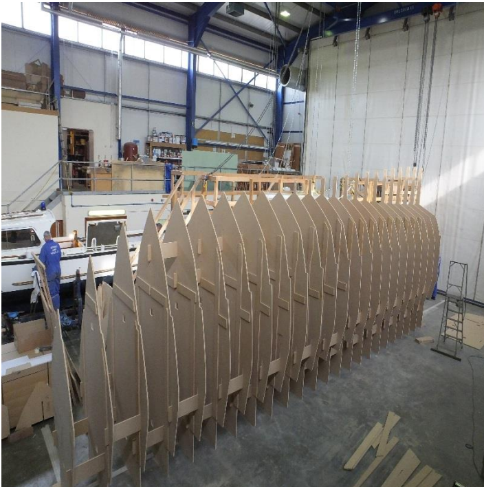
Medium Density Fibreboard station 2 -26 positioned
